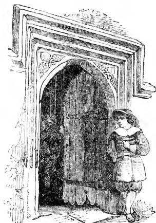
Belfry Porch, Elstow.
